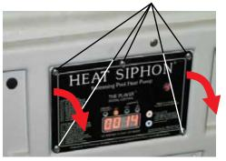
Remove Screws and tilt door forward
